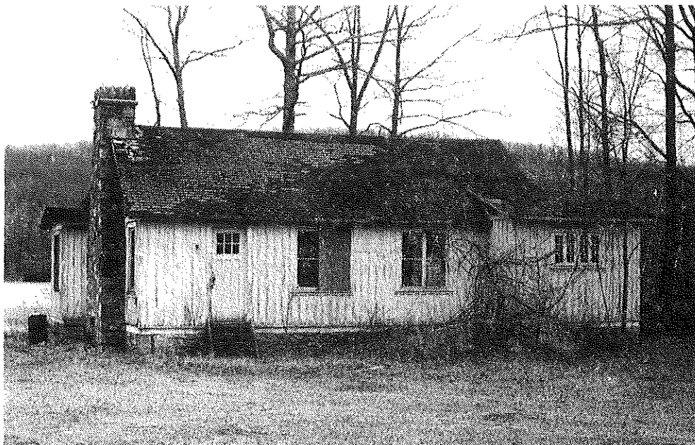
Figure III-3 - The Lodge (1981 Photo)
