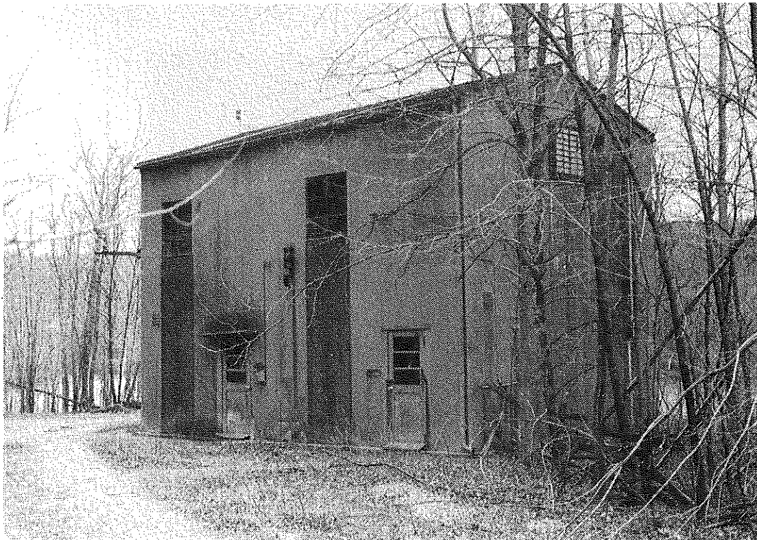
Figure III-10 - Shield Mock-Up Building (1980 photo)
